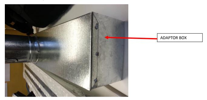
3. MARK HOLES TO BE MADE INTO THE ADAPTOR BOX TO ENSURE A SECURE FIT FOR THE VENT USING THE RECESSED HOLES IN THE VENT AS A GUIDE. TWO PEOPLE MAY BE REQUIRED FOR THIS.
