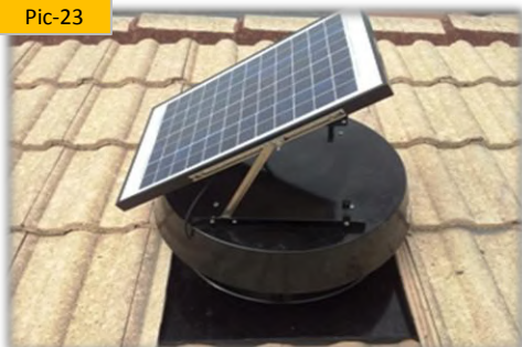
The installation is now complete.
