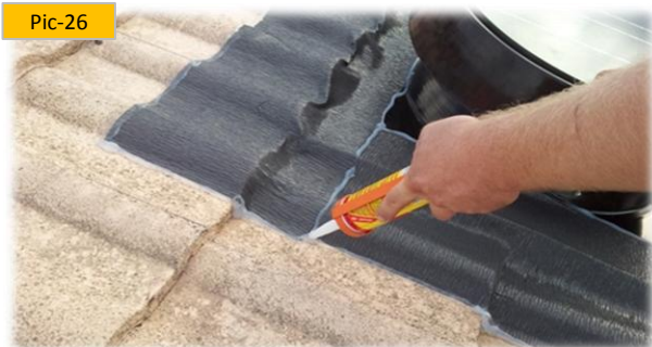
Pic-26 Continue sealing all edges and overlaps with silicone until complete.
