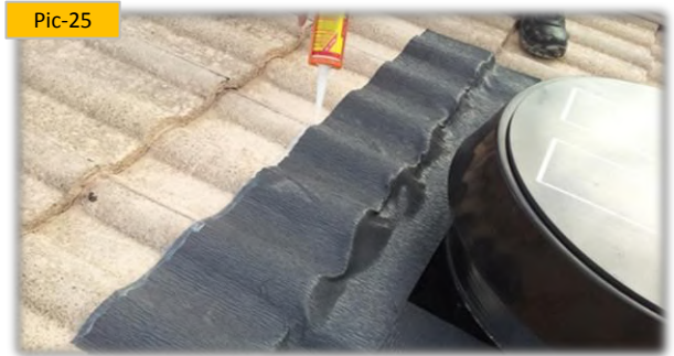
Pic-25 Now that the flashing is complete, you need to run a seal of silicone along all the edges of the flashing including any overlapping points.
