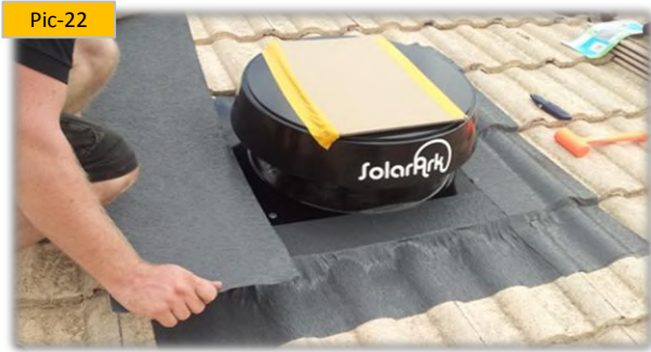
Pic-22 Attach the other side piece of flashing and conform to the shape of the tiles.
