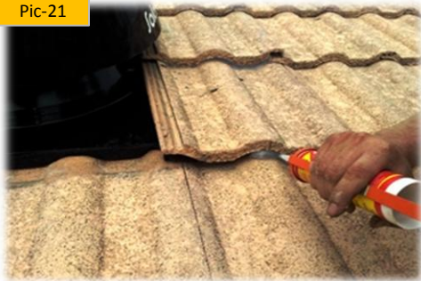
Sealing minor gaps.
