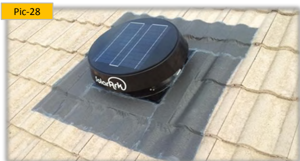
Pic-28 The flashing can finally be painted to match the roof colour if required.
