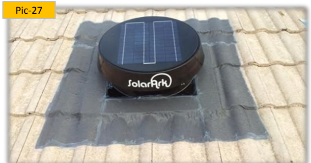
Pic-27 The final stage is to make sure that you have removed the cardboard cover from the solar collector. Once this is done the SolarArk solar roof fan will start working provided the temperature inside the roof is above approx 24 °C and the solar panel is exposed to medium-high sunlight.
