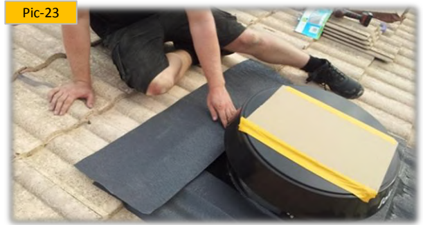
Pic-23 Finally attach the last flashing to the top of the solar fan base plate and tiles. Conform to the shape of the tiles.
